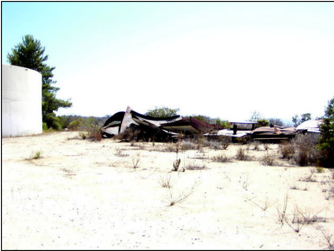
Photograph 3: View toward Avocado Flats candidate location, facing southwest.
